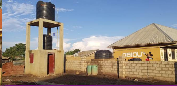
New water system at the P4T primary school
