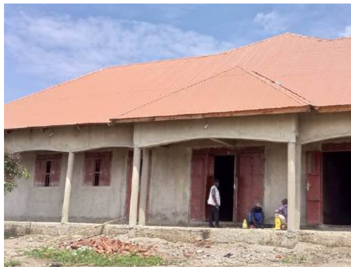
Vocational Skills Centre under construction
